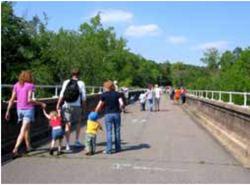
Everyone loves walking the old pedestrian bridge over the Haw in Bynum, at the Haw River Festival
