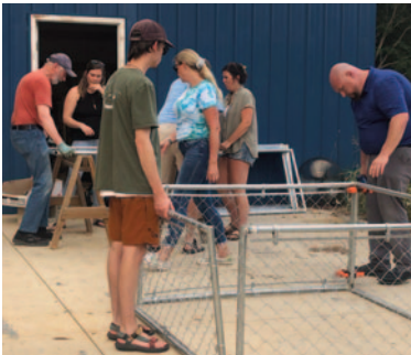
Volunteers help build a Trash Trap.
