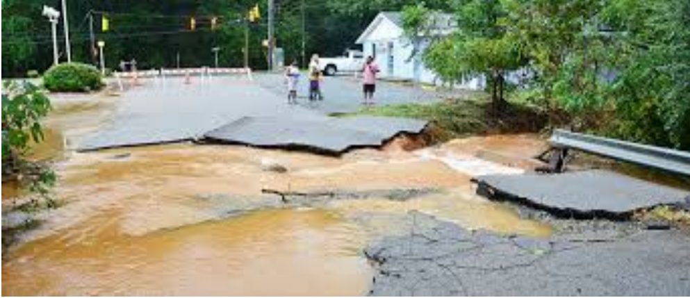
Photo of Robeson Creek tributary flooding damage, resulting in road closures for over six months and thousands of dollars from Pittsboro town budget and FEMA. Photo by Chatham News and Record 2
